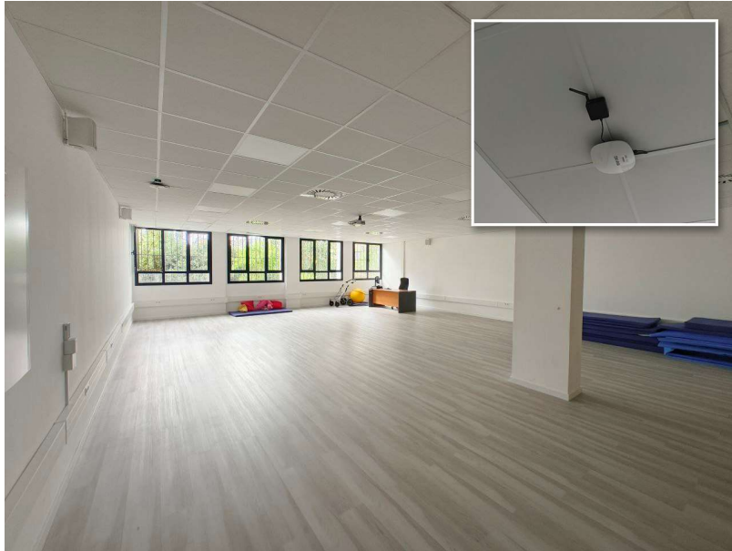
Sensor-equipped teaching space: the IoT network watches over environmental conditions by reusing the HPE Aruba access points already present on campus (detail).
