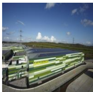
Morrisons Distribution Center (UK)
