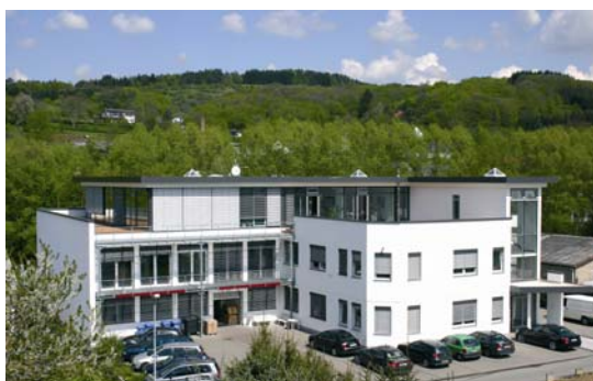
Fig. 5: Office Building with LON/EnOcean Technology
