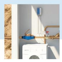
Application For manually or remotely controlled closing and opening of a water pipe in buildings in response to an event message from the water sensors WaterSensor eco or WaterSensor con.
