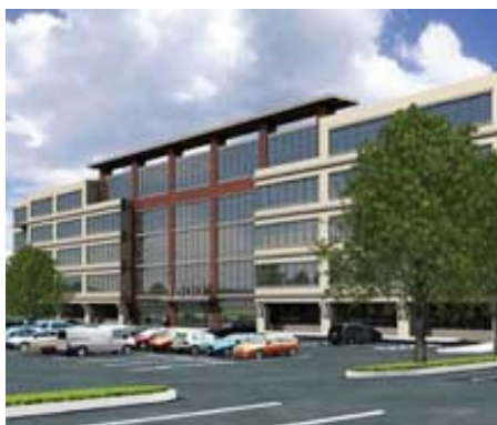
Picture 4: Office Building 1,000 Continental, King of Prussia, PA with EnOcean enabled wireless sensors
