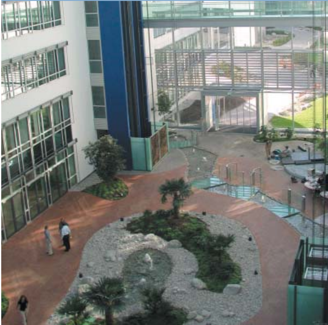
The fully-glazed courtyards also ensure that the staff working in aviva MUNICH enjoy a pleasant environment.
